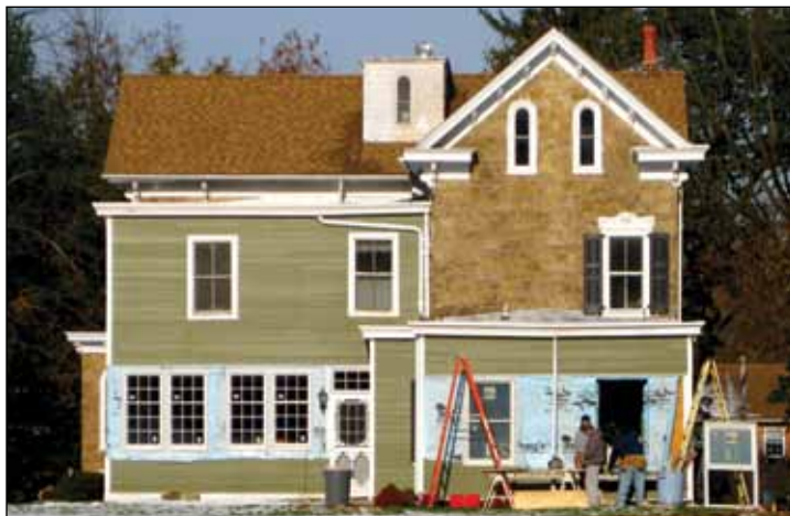
This historic building has a wide variety of old and new windows.
