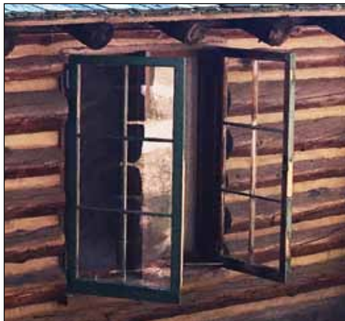
These historic windows have full screens inside the casements, which are hinged to open easily to facilitate window operation.
