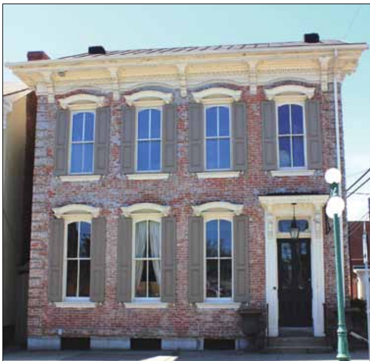
Can you see the storm windows on this historic house? The left three windows on the second story have exterior storm windows, while the others do not.
