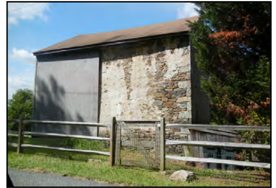
South elevation of Half Barn near Birchrunville.
