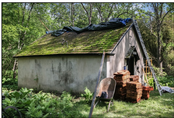
Crystal Diamond Springhouse with deteriorated roof. Photograph by James B. Garrison.
